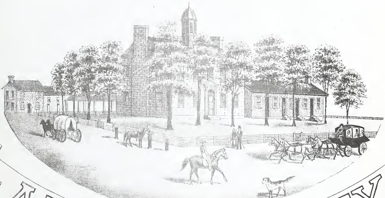
Built by Gov. Thomas Worthington of Ken. 1811
