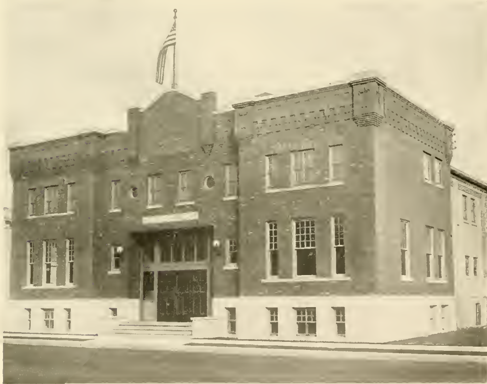
NEW ARMORY, CROOKSTON
