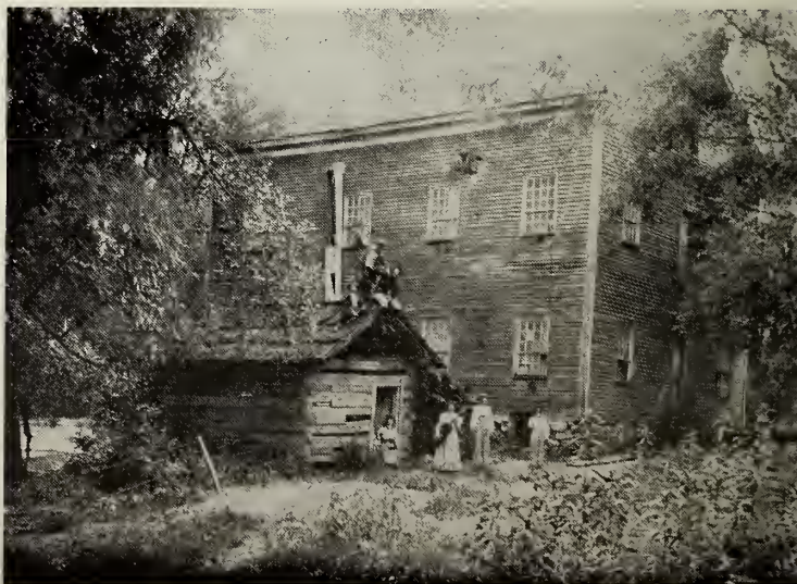
Old mill located at the north edge of town, just east of U.S. 35.
