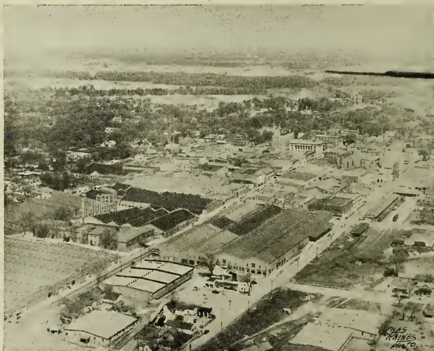
Aerial View of Business Area of Wilson
