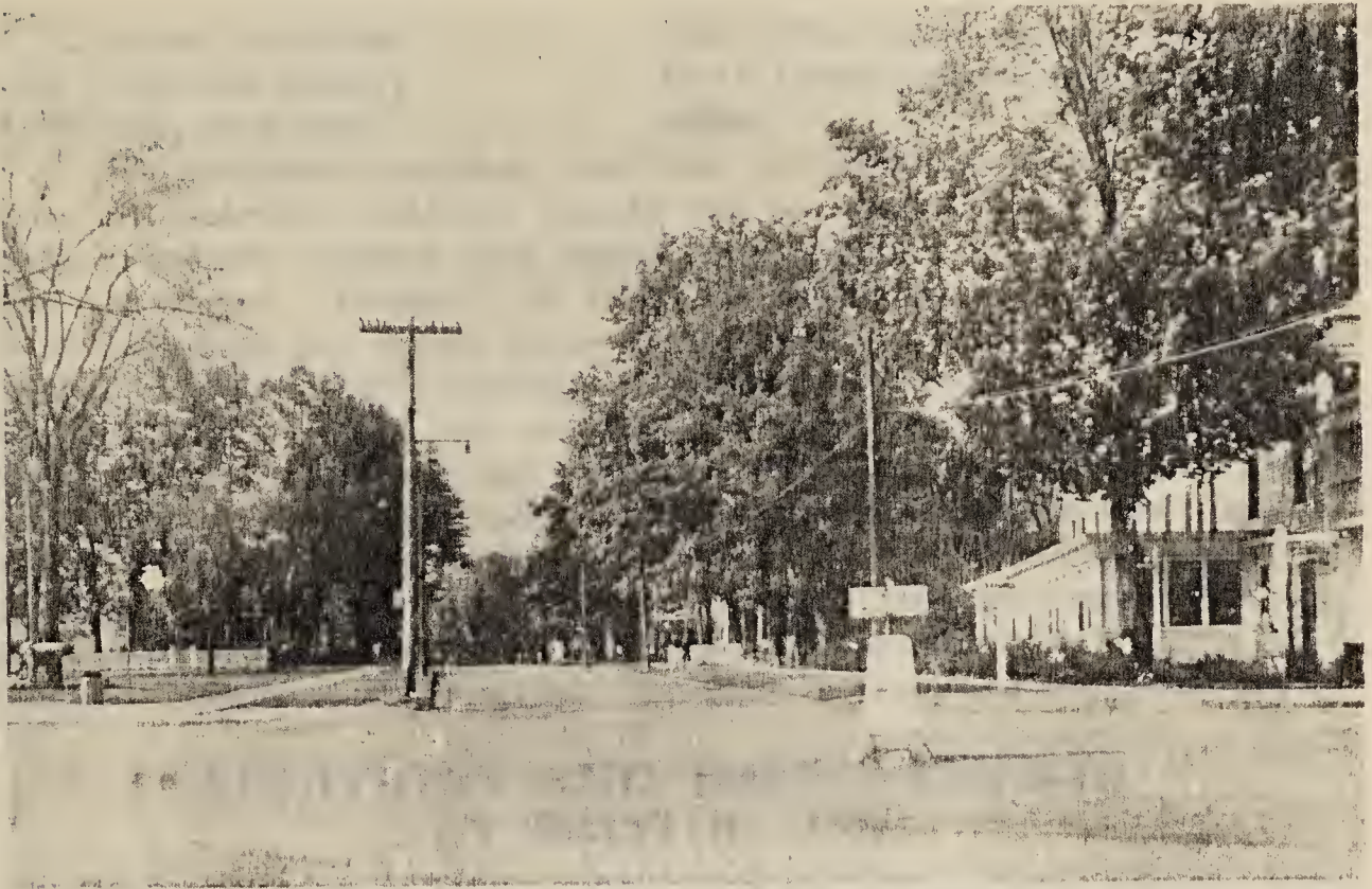
North Street Showing Corner Of Park At Left
