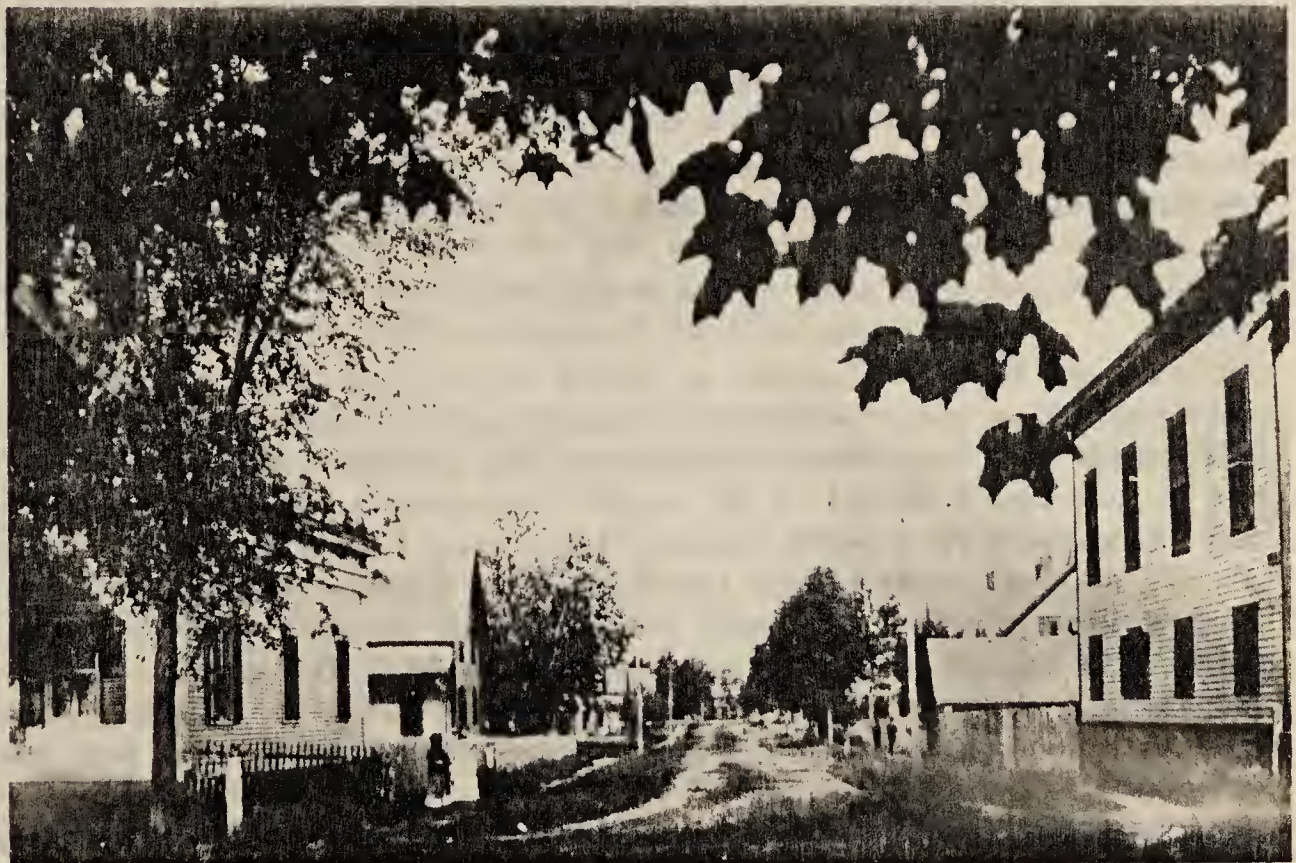
Church Street Looking West Methodist Church (Before Remodeling) At Right
