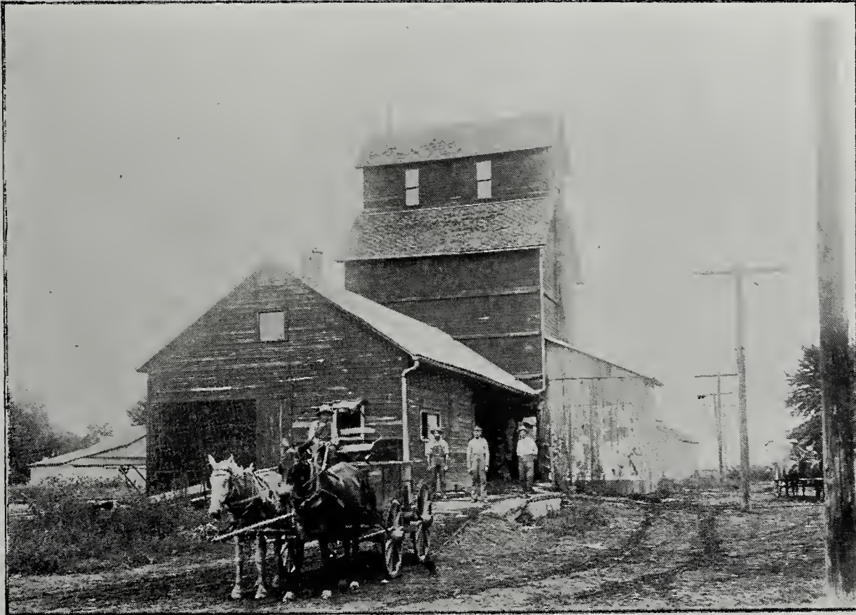
RAYBURN'S GRAIN ELEVATOR, GREEN RIDGE, MO.
