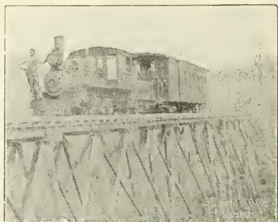
P. & H. Train on the Trestle.
