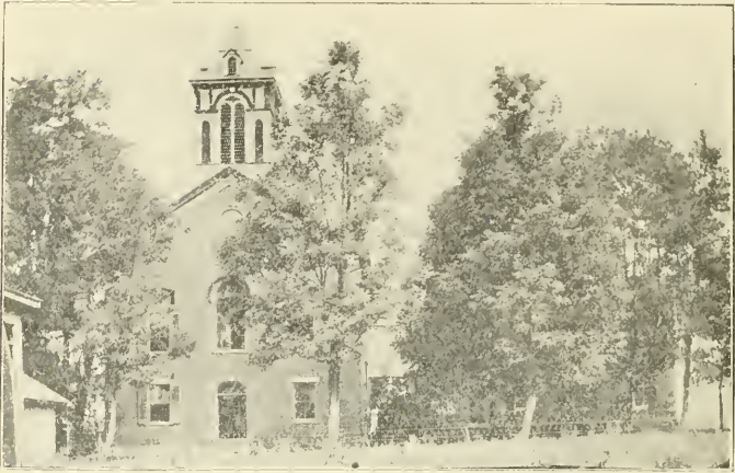
The Court House with the annex.
