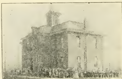
Harrisville School Building.
