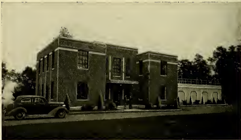
WATER PURIFICATION PLANT
